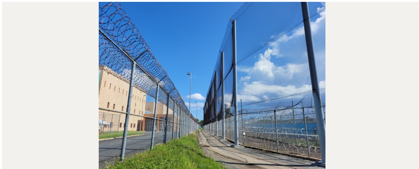
Security perimeter netting — Bayamón, Puerto Rico Department of Corrections.
