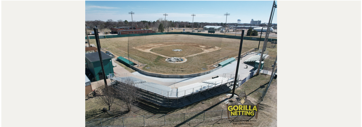
Cable-suspended tie-back backstop netting at Bill Wood Field — North Platte, NE.
