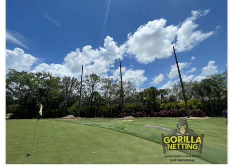
Eagle Creek Golf Course Pole & netting system.
