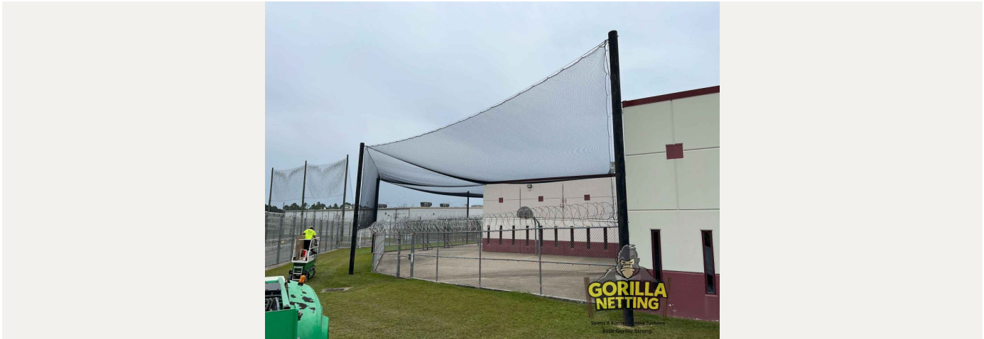
Overhead contraband netting installation at a high-security correctional facility.
